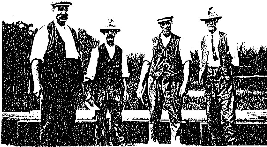
The men building the bungalows - from the left:-
